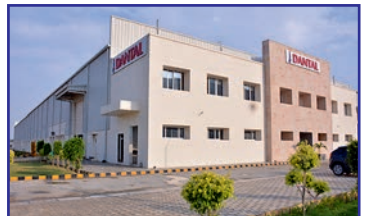
Cylinder Plant, Ghiloth, Rajasthan
